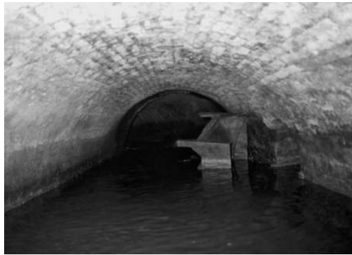
Figure 14. Brick culvert sprung from stone walls to the south of the Lower Furnace site. The tunnel visible in the right-hand (eastern) wall, adjacent to the upturned crate, is the tailrace to the grinding wheels returning to the main watercourse, fossilised in the culvert structure (Photograph by OnSite Surveys, reproduced courtesy of the Borough of Telford and Wrekin).
