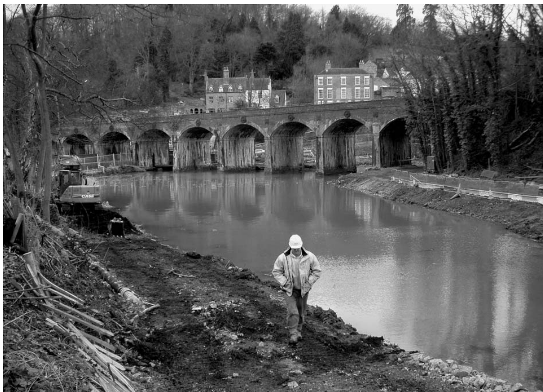
Figure 16. Upper Furnace Pool after the second phase of desilting works in 2005. The central haul road has been removed, and operations were undertaken along the road along the northern side of the pool (Photograph by Paul Belford).
